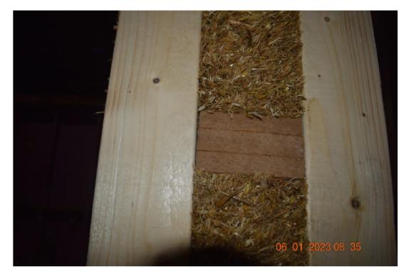
Photo No. 2 Straw insulation between the load bearing studs.
