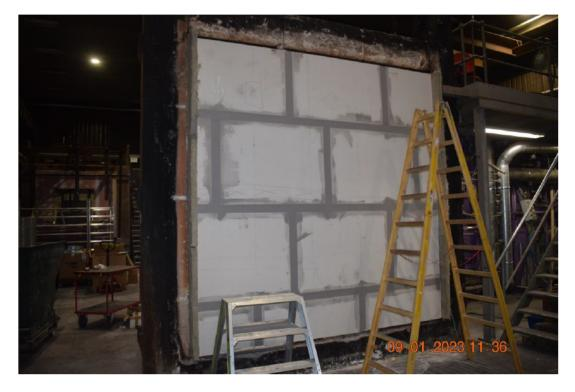
Photo No. 10 Spackle applied over the joints of the gypsum board.
