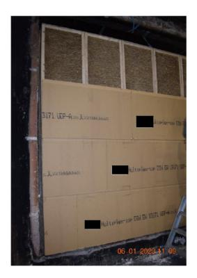
Photo No. 6 Mounting of wood fibre board, exposed side.
