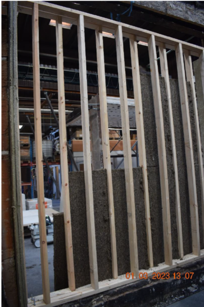
Photo No. 1 Timber frame of specimen, with seaweed insulation.
