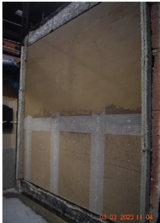
Photo No. 5b Test specimen with clay plaster being added
