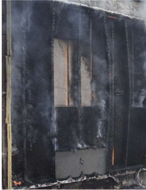
Photo No. 16 Test specimen doing disassembly
