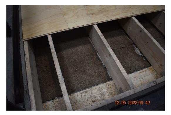
Photo No. 13 Plywood as top layer
