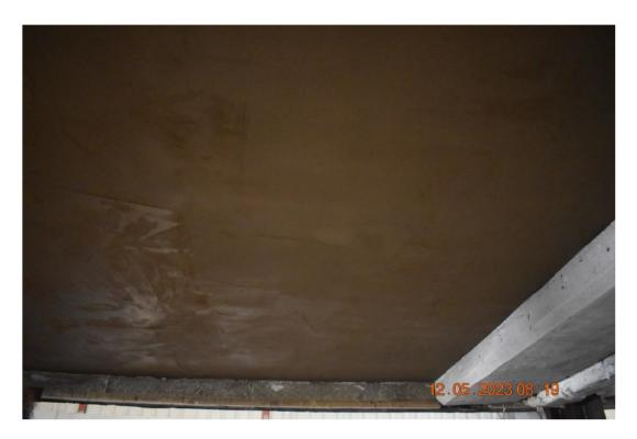
Photo No. 12 Clay rendering during mounting
