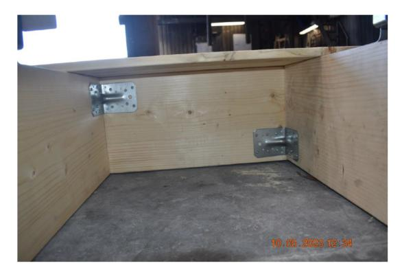
Photo No. 5 Timber joist connection.
