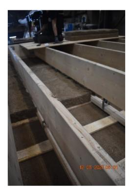
Photo No. 11 Insulation during installation
