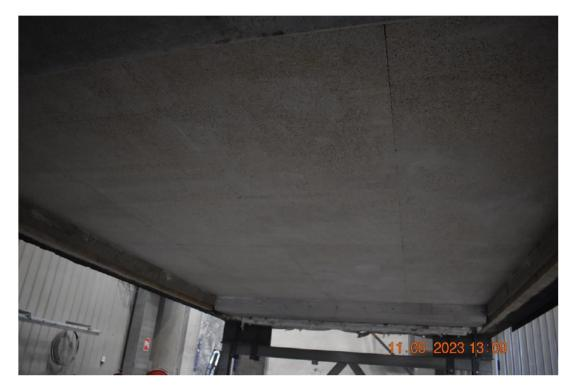
Photo No. 9 Hemp boards mounted to the clay boards.
